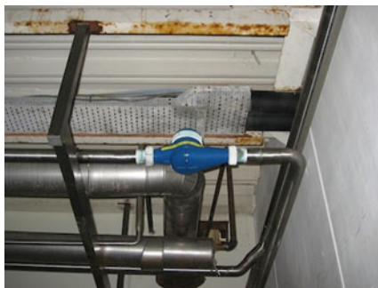
One of the new water meters installed.
