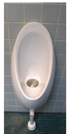
Example of a waterless urinal.
