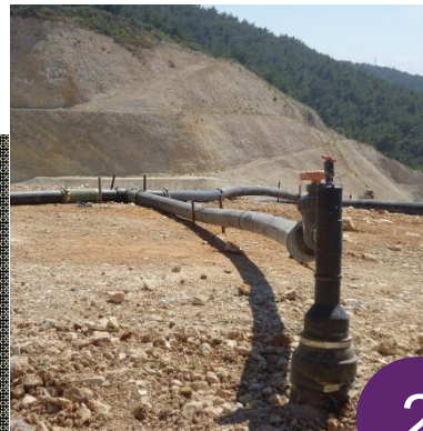
GAS WELL HEAD CONNECTED TO NETWORK
